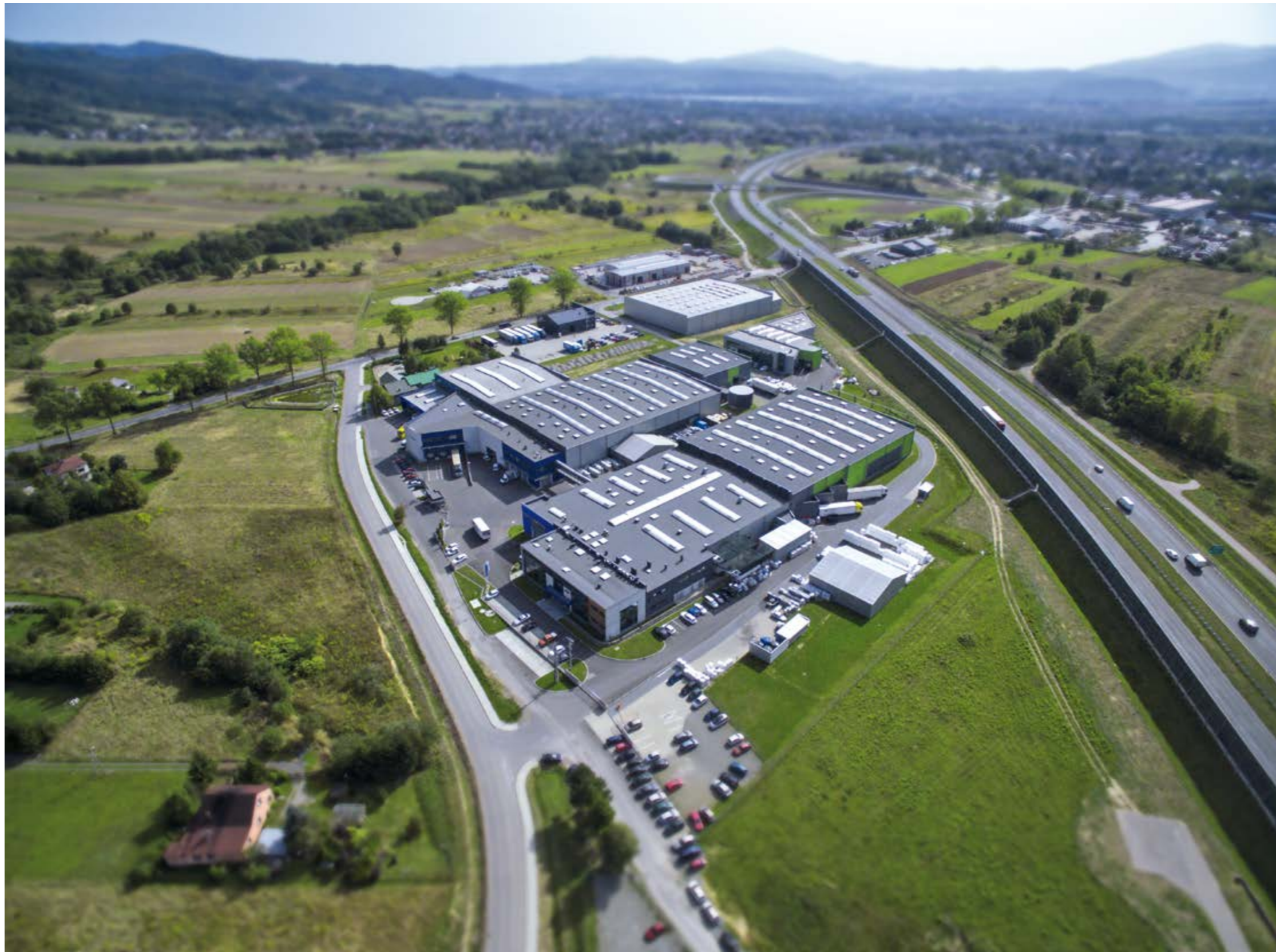
Rybarzowice - headquarter (production & warehouse)
