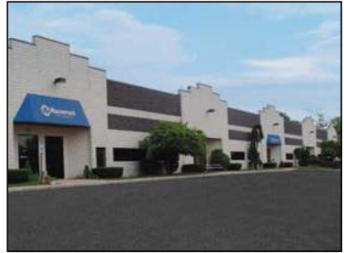
European Sales Office and Warehouse
